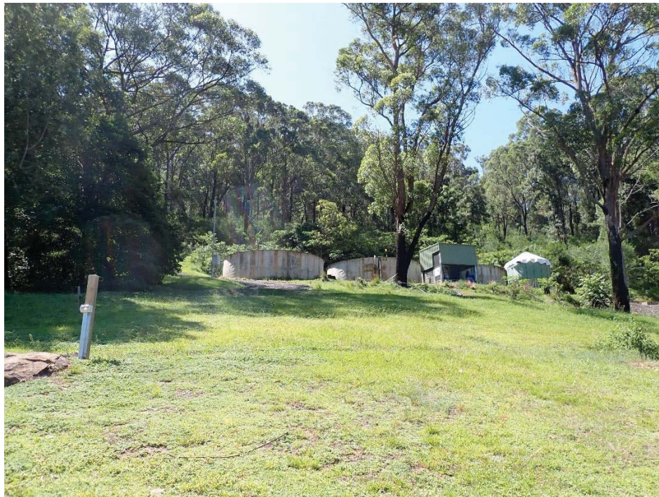
Photograph 06: Existing 3 x 100,000L Concrete water tanks
