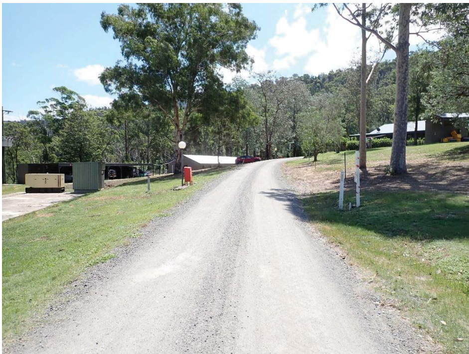
Photograph 06: View north of the existing internal access road to be upgraded
