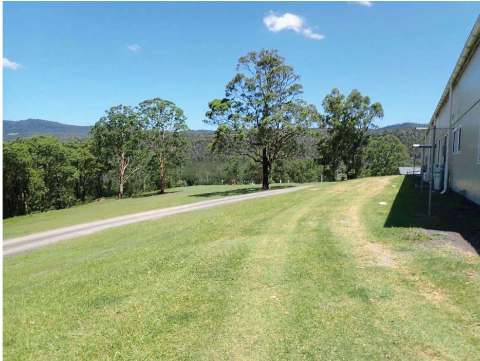
Photograph 05: View of the existing access to be upgraded adjacent to the proposed Building D2 (Existing building to be demolished)
